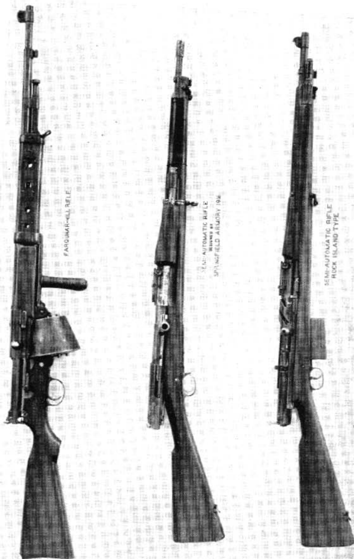
Left: Farquhar-Hill rifle, tested at Springfield Armory in 1917. Middle: Gas operated semiautomatic rifle designed at Springfield Armory, 1916. Right: Gas operated semiautomatic rifle designed at Rock Island Arsenal, 1916.
