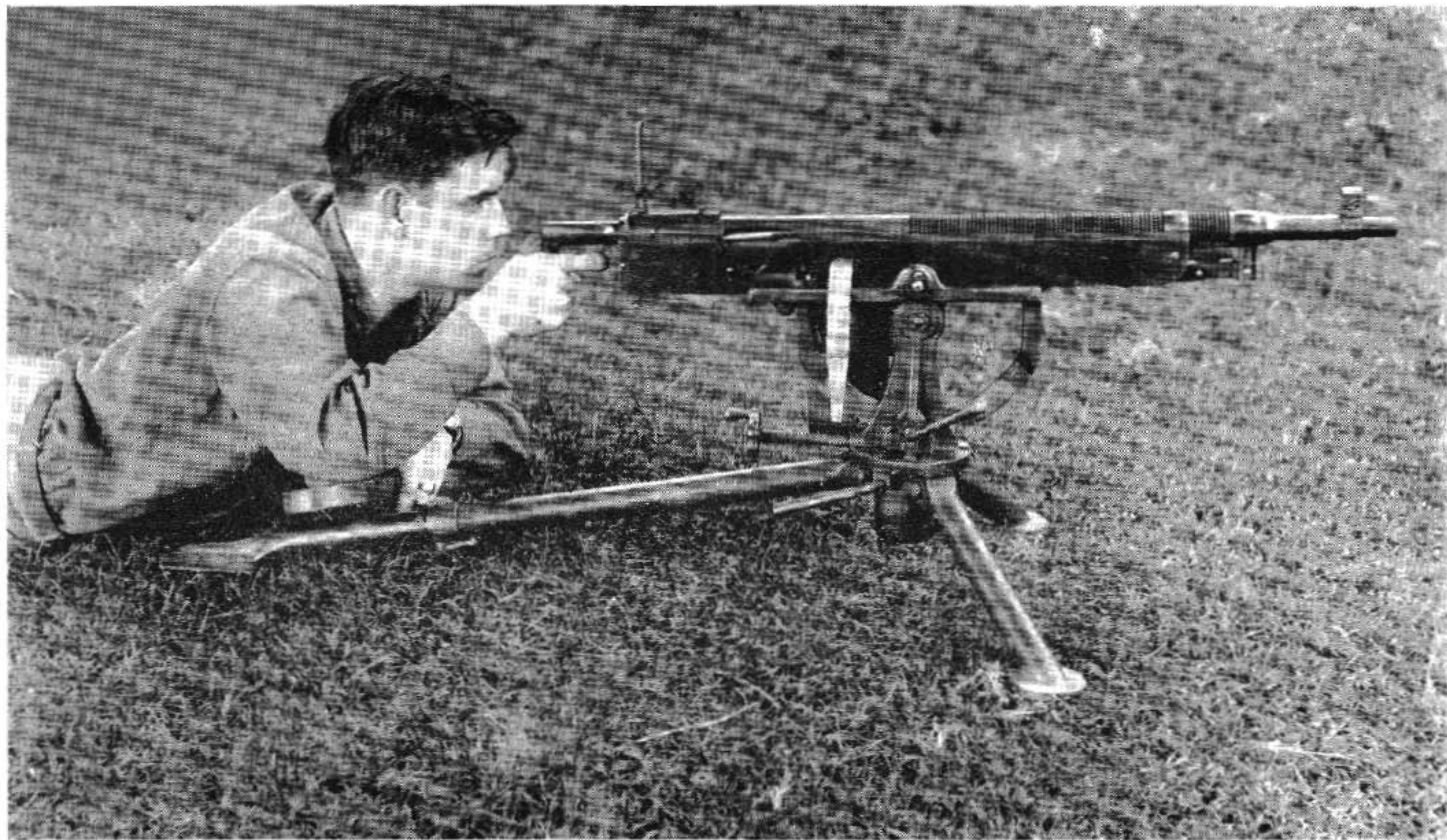
Colt machine gun, invented by Bowning in 1889. The gas passing through a port about six inches behind the muzzle impinged on a lever pivoted under the gun, swing it downward and backward to actuate the mechanism. The present author is shown firing one of these guns in 1917, when they were being made for the Russians by Marlin-Rockwell.
