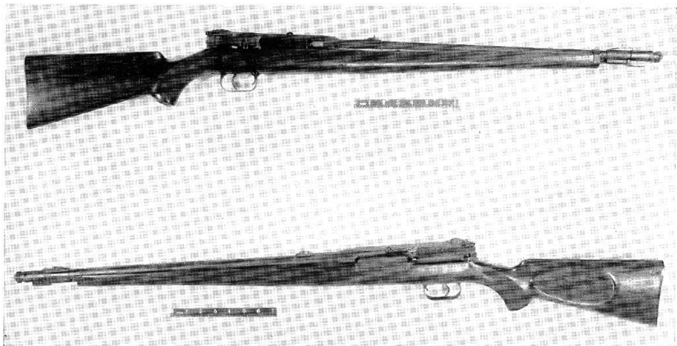
Heinemann semiautomatic rifle, made for the 7.92mm German service cartridge, captured in Germany during World War II. This is very similar to the .276 model of this gun that was tested in Aberdeen Proving Ground in 1929.
