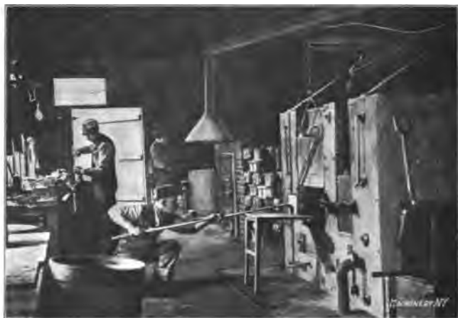
Fig. 39. Gear Case-hardening Room in the Premier Factory
