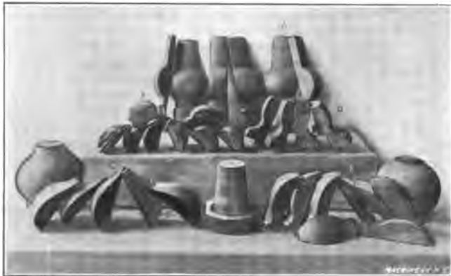
Fig. 29. Sectional Chucks made from Wood
