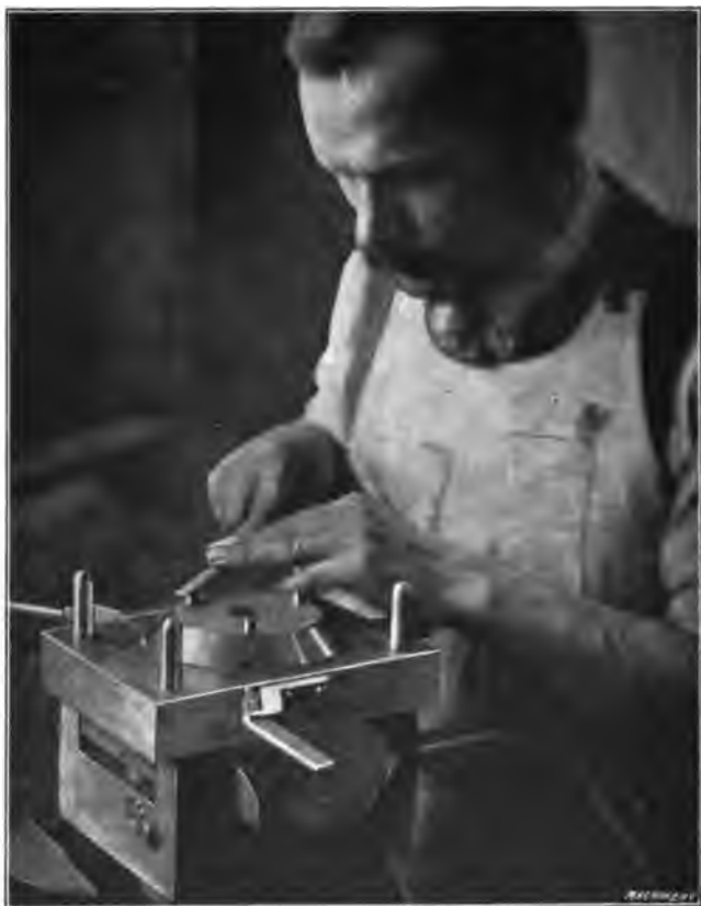
Fig. 41. Fitting Ejector-pins
