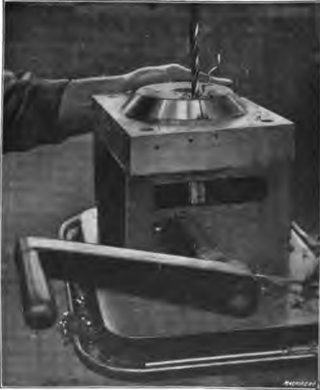
Fig. 40. Drilling the Ejector-pin Holes
