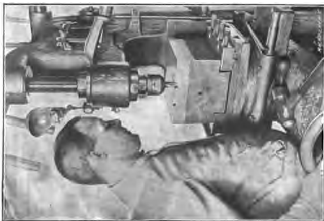
Fig. 94. Milling the Gate
