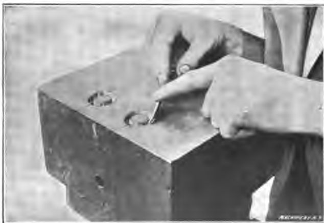
Fig. 17. Scraping Out the Impression
