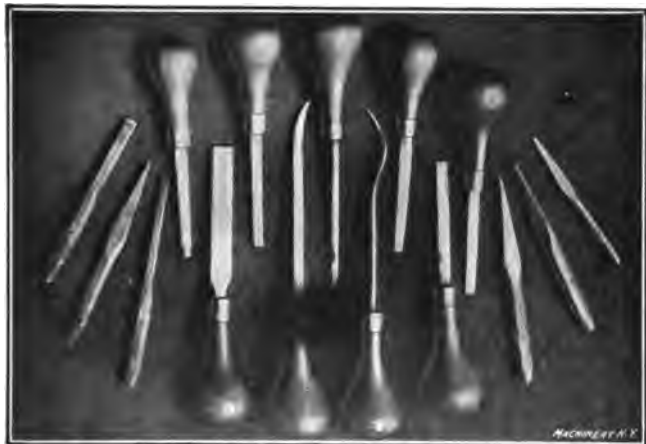
Fig. 14. Chisels and Scrapers used in Die Sinking
