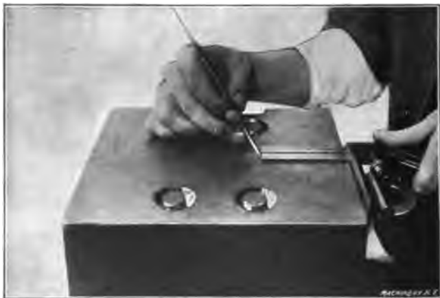
Fig. 5. Laying out the Dies: Transferring a Line from One Die to the Other of a Pair
