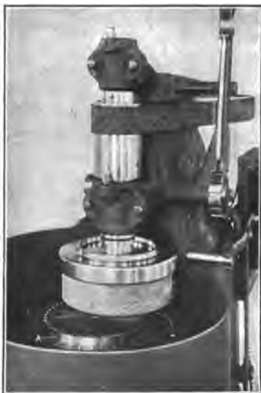
Fig. 28. Grinding Side of Saw Concave
