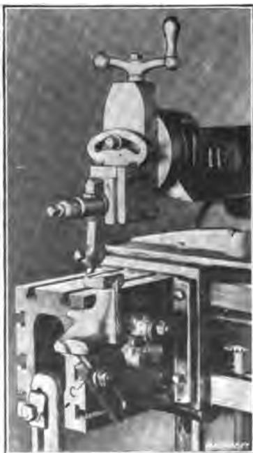
Fig. 45. Casting of Irregular Shape bolted to Side of Table
