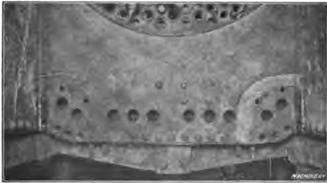
Fig. 4. The Completed Weld with Sections of the Throat Sheet replaced
