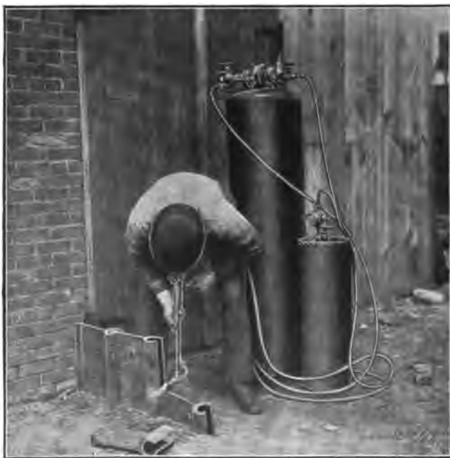
Fig. 6. Cutting Off Steel Sheet Piling with Oxygen Cutting Torch showing Portable Apparatus
