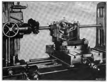
Fig. 89. Boring Differential Gear Casing
