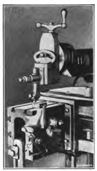
Fig. 45. Casting of Irregular Shape bolted to Side of Table
