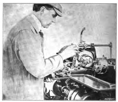
Fig. 21. Operator setting a Circular Form Tool
