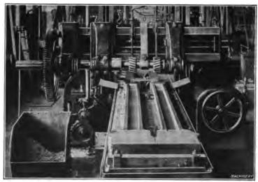
Fig. 32. Channeling the Sides of Locomotive Main-rods on Horizontal Machine it is counterbalanced by weights attached to wire ropes that pass over the pulleys at the top of the housings.
