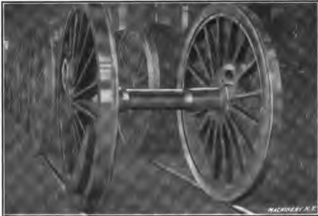
Fig. 30. The Wheels ready for the Crankpins
