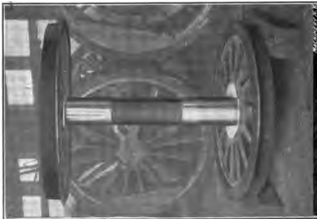
Fig. 26. Shrinking the Tires onto the Centers
