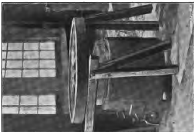
Fig. 18. Pre-heating the Wheel Center while Melting the Bronze for the Hub Liner
