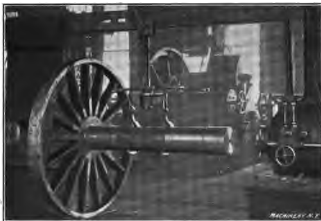
Fig. 23. Pressing the Axle into the First Wheel
