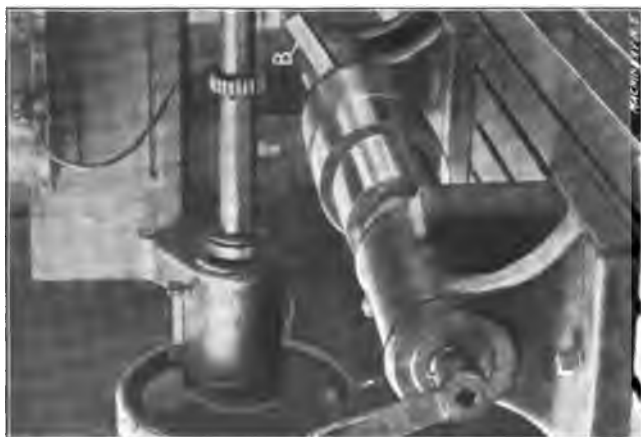
Fig. 12. Keyseating the Crankpin in the Horizontal Miller.
