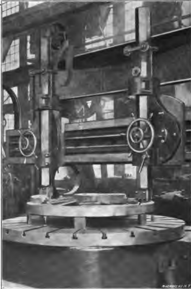
Fig. 19. Boring and Turning the Wheel-center
