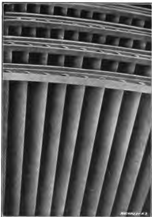
Fig. 49. Rows of Blading of Allis-Chalmers Turbine
