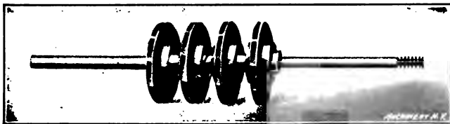
Fig. 17. Impellers of Turbine Pump
