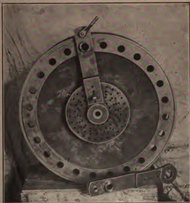
Fig. 45. Adjustable Flange Drilling Jig
