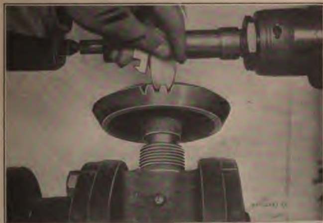
Fig. 14. Testing Accuracy of Settings for Approximating the True Tooth-form
