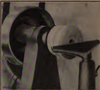
Fig. 24. Turning the Seat for the Hub
