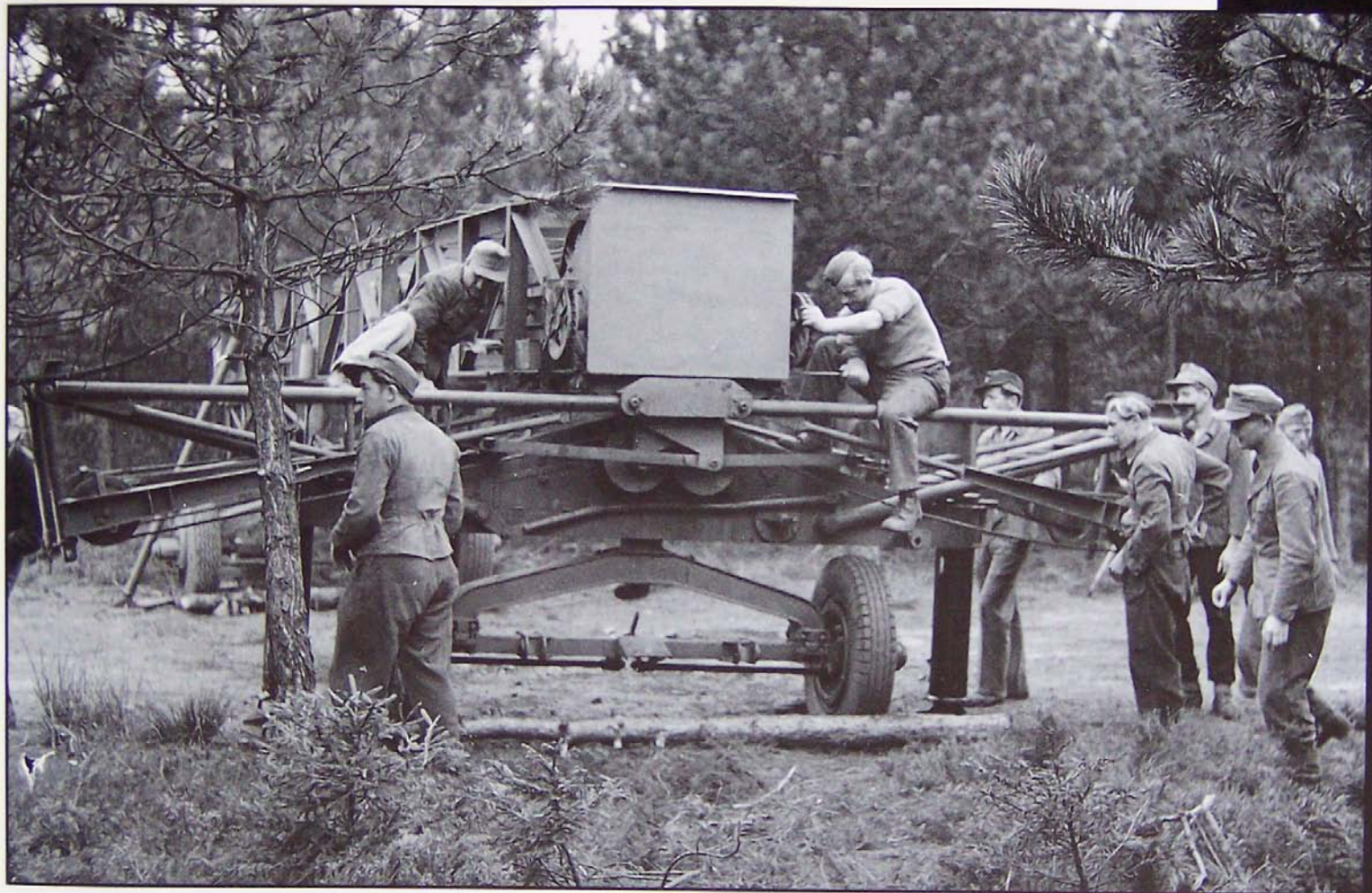
With the folded end frame turned sideways to the cross piece, the crew could then raise the crane structure. The scissors design was light weight and very strong. The cable and pulley system was the simplest way to move the scissors to raise (or lower) the entire crane. After adjusting the cables and pulley system, the crew carefully began lifting the crane, making sure the two ends were raised evenly together. The large jack struts were adjustable and were locked in place before the crew raised the gantry. Stabilizing the crane was very important, as the heavy loads could cause an unstable crane to fail. (IWM)
