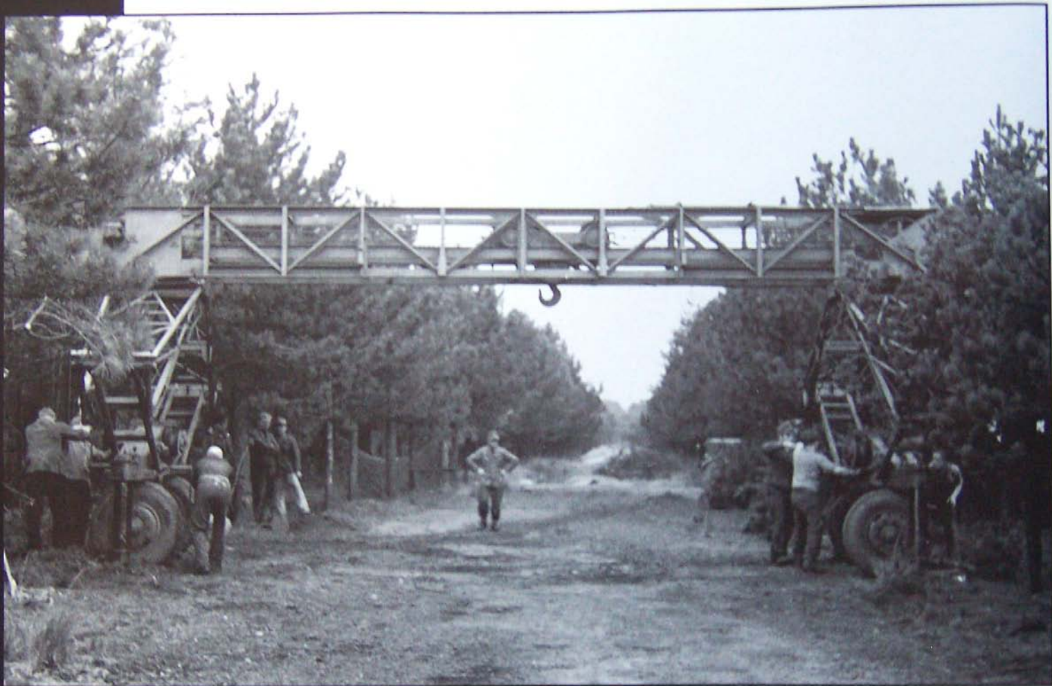
The 15-ton gantry crane was a large structure, long enough to straddle two railroad tracks to transfer loads from one train to another or to a truck or wagon parked next to the track. The motorized bogie truck and lifting hook ran transversely along the gantry, allowing loads to be moved side to side. Here, the crew had raised the gantry about half way, tightening the cables on the tower frames to lift the cross piece to its full height. Because of the size of the V2, the gantry crane needed as much ground clearance as possible. (IWM)
