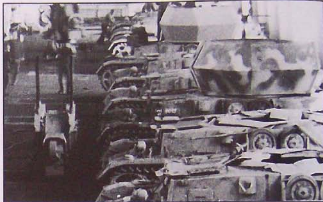
Above and below: The large assembly hall of Ostbau in Sagan. More than 10 Wirbelwind in various stages of production wait for completion. It is evident that different versions of the Pzkw IV were used. In the foreground of the lower photo, two late Ausf. H can be seen; the hulls farther in the back are possibly Ausf. G or early H. Note that early style drive sprockets were used. The empty brackets for the side skirts are visible, too. The hull with the number 4015 is already fitted with a turret. The typical Ostbau camouflage was also applied. The 2 cm Flakvierling 38 (Panzerabwehrung) waits for installation. Photos v. Seherr-Thoss.
