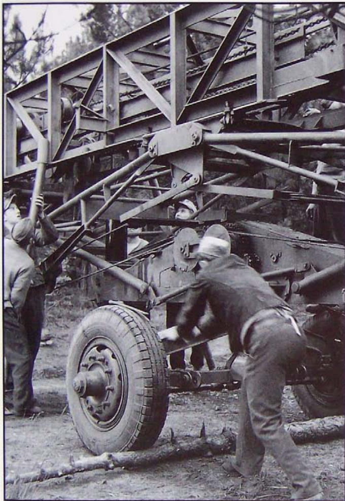
Left: Erecting the gantry crane took a number of men, as the process of unfolding the support structures had to be done manually. With the road wheels blocked against a tree trunk, the crew began the task of erecting the crane. Time was of the essence in the last months of the war, due to Allied planes, but in fact, the great difficulty in spotting a V2 being prepared for launch made this a fairly safe procedure. The complex scissors arrangement of tubes and struts had to extend and retract reliably and quickly, but also had to support the weight of the gantry overhead frame and of the load being carried. (IWM)
