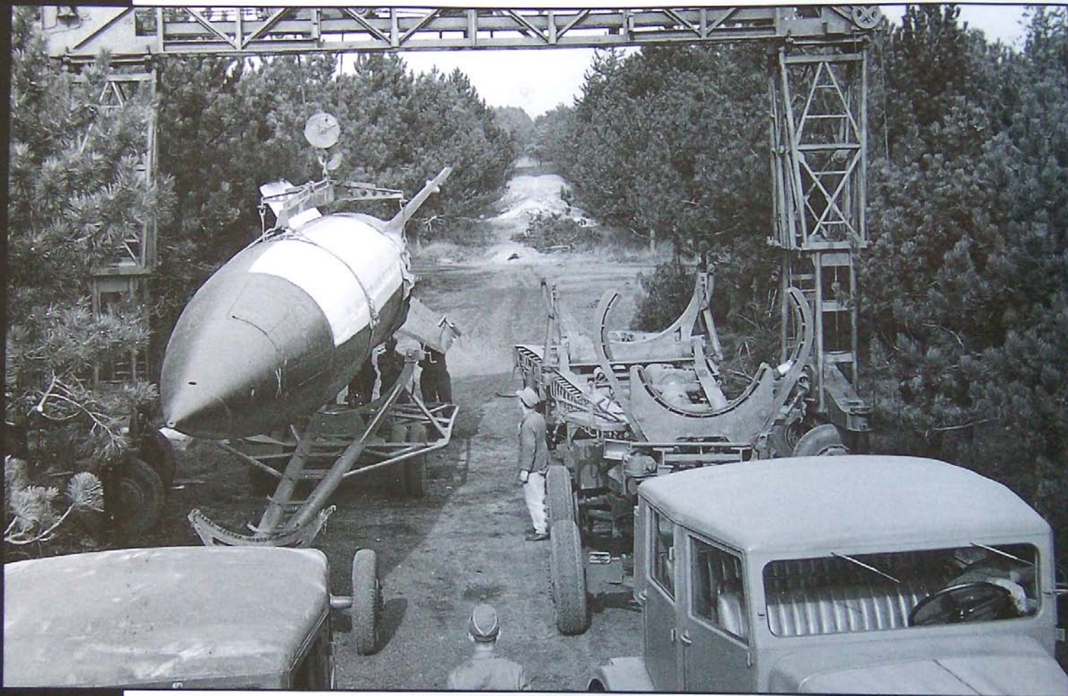
The missile was lifted from the Vidalwagen trailer (left) and moved to the other side of the gantry to be loaded onto the MeiBlerwagen. As seen here, the Vidalwagen had a simple tubular frame intended only for transporting the missile. The MeiBlerwagen was heavier and much more complex, designed to transport the missile to the launch site and then launch it. The MeiBlerwagen also supported the V2 during fueling, which could be done only at the launch site. (IWM)
