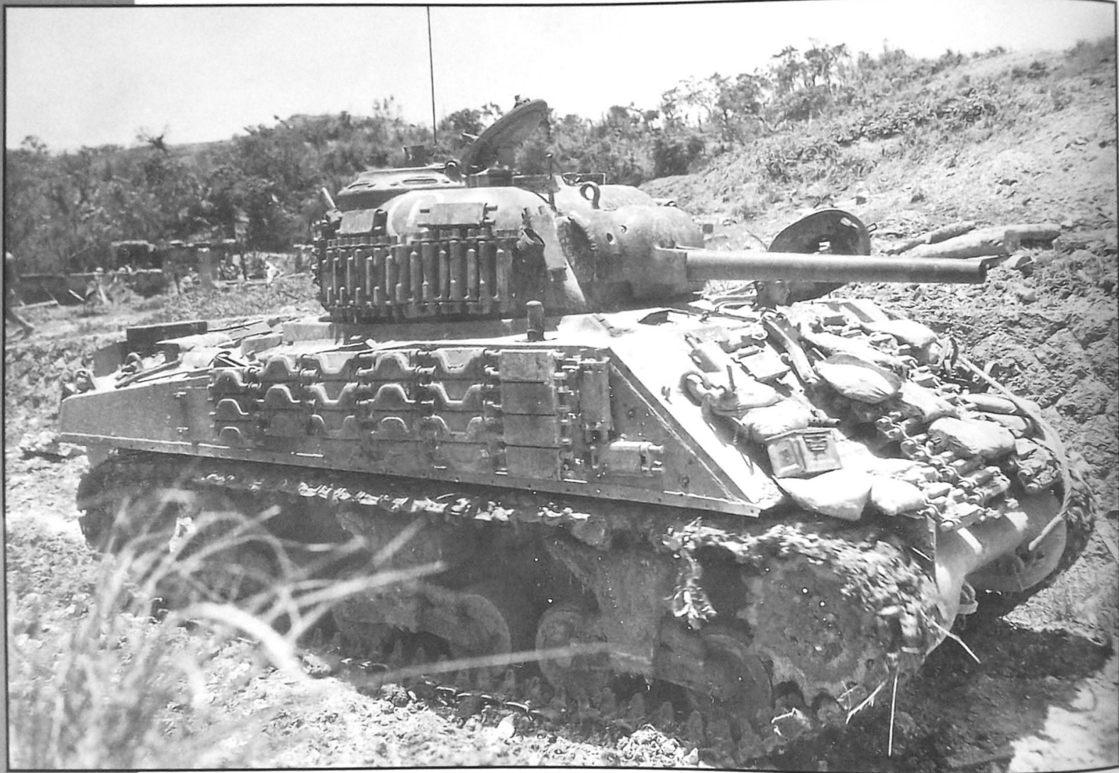
A late M4A3 moves forward to assault Oroku Village on 7 June 1945. This is a tank of 2nd Platoon, B Company, 6th Tank battalion. This unit was part of the landing on 4 June at the Oroku Peninsula. This tank is a fine example of the late M4A3 with its commander's cupola, (apparently) solid road wheels and drive sprocket, and enlarged forward hatches. The hull of the tank is liberally covered with spare
