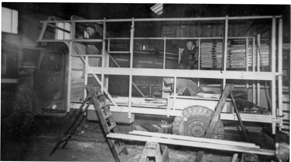
An interesting photo depicting the framework construction on a Bedford 3-ton cab and chassis. This is the workshop of J C Clark Ltd of Greenside, London.
