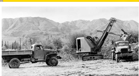
Below: Most of the gravel used for surfacing along the Alcan Highway was obtained from glacial deposits found alongside the roadway. (US Library of Congress)
