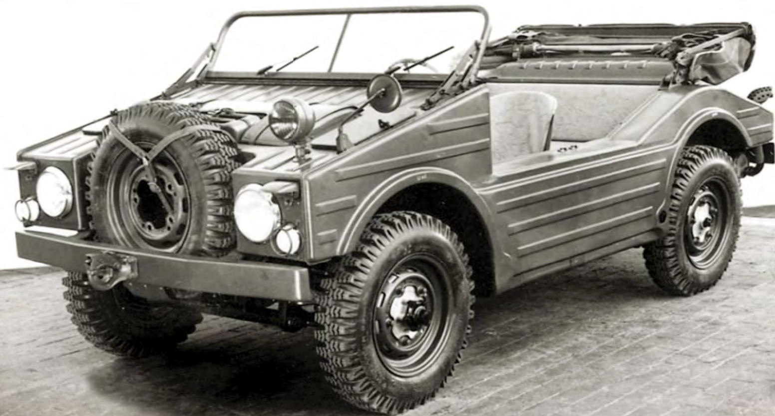
Above: The military variants came with NATO hitches front and rear.
