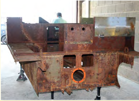
A new drop-down panel for the rear of the crew compartment was fabricated.
