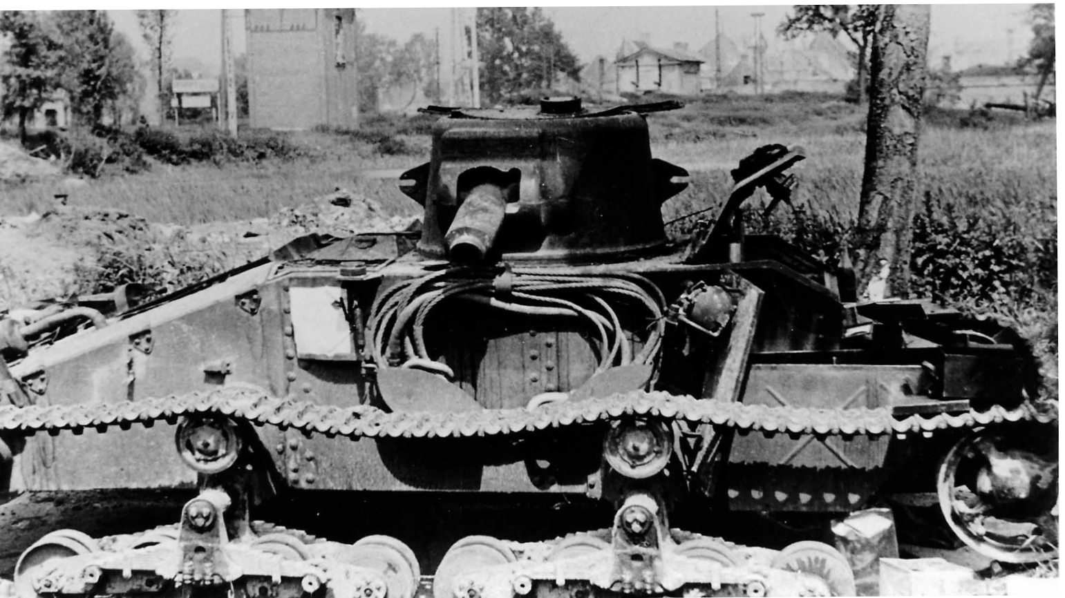
An A11 Matilda 1, abandoned near Arras. These tanks formed the main strength of 1st Army Tank Brigade but they were almost useless for fighting other tanks.
