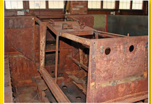
The skeleton of the engine housing stripped of its panels.
