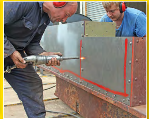
Hot riveting the replacement right-hand panel.
