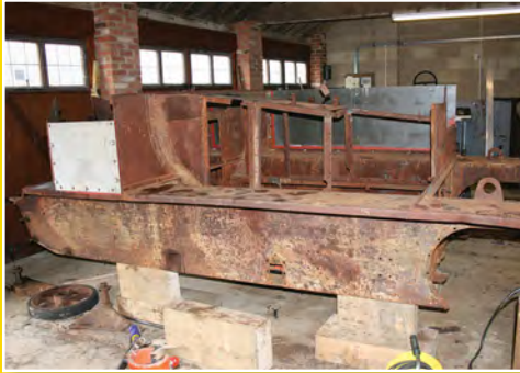
A replacement for the holed left-hand forward panel is temporarily fixed prior to riveting.
