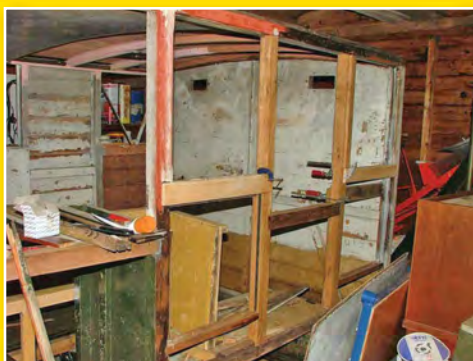
This side of the body was crashed in but Bob managed to keep as much of the original woodwork as possible.
