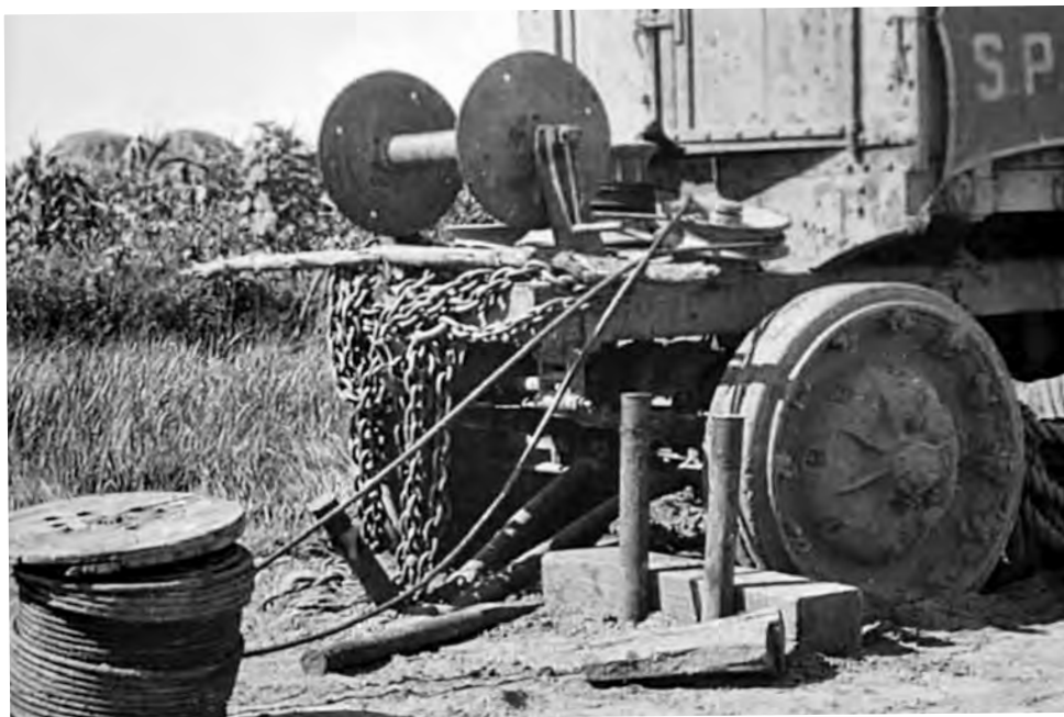
With a heavy winch powered by the Wisconsin engine and the back wheels chocked into place this Militor is hauling out other trucks stuck in gelatinous mud.
