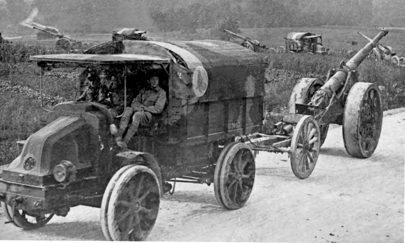
Above: One of the trucks used as an inspiration for the Militor was the French Latil TAR. This truck had been designed in 1913, had the capacity to tow 12 tons and like this one was used by the French army for hauling heavy artillery.
