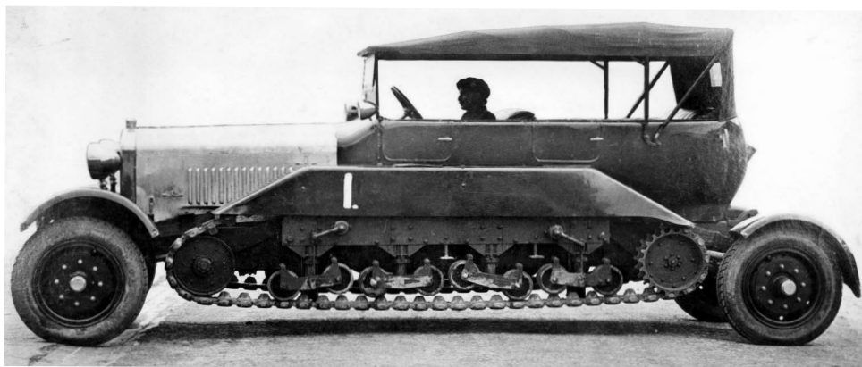
The Vickers-Wolseley wheel-cum-track staff car in wheeled mode, referred to officially as a Reconnaissance Car.
