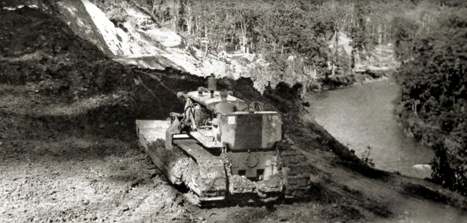
Caterpillar D8 of Company C at work on the Ledo Road near Loglai, in the Patkai range (1880th Aviation Engineer Battalion).
