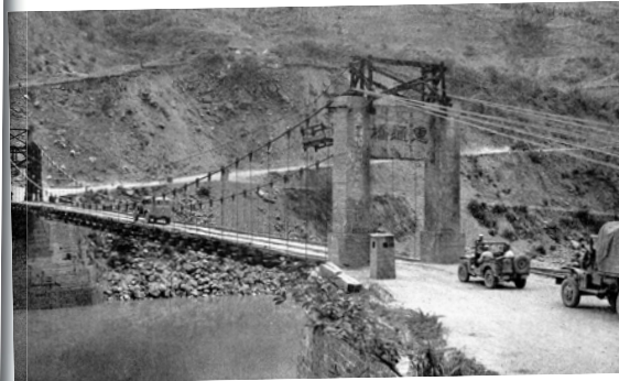
Above: A Dodge WC-53 Carryall is crossing the splendid suspension bridge over the Salween River, followed by a Jeep and a GMC (1880th Aviation Engineer Battalion).
