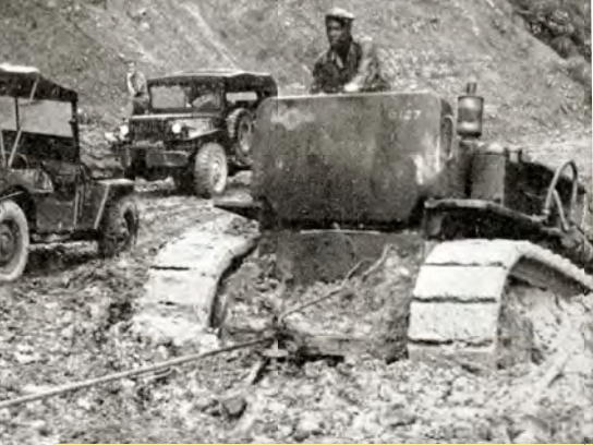
Above: Caterpillar D8 sunk in the mud (1880th Aviation Engineer Battalion). Right: Mechanics work continuously to repair equipment; here an International TD 18 (1880th Aviation Engineer Battalion).
