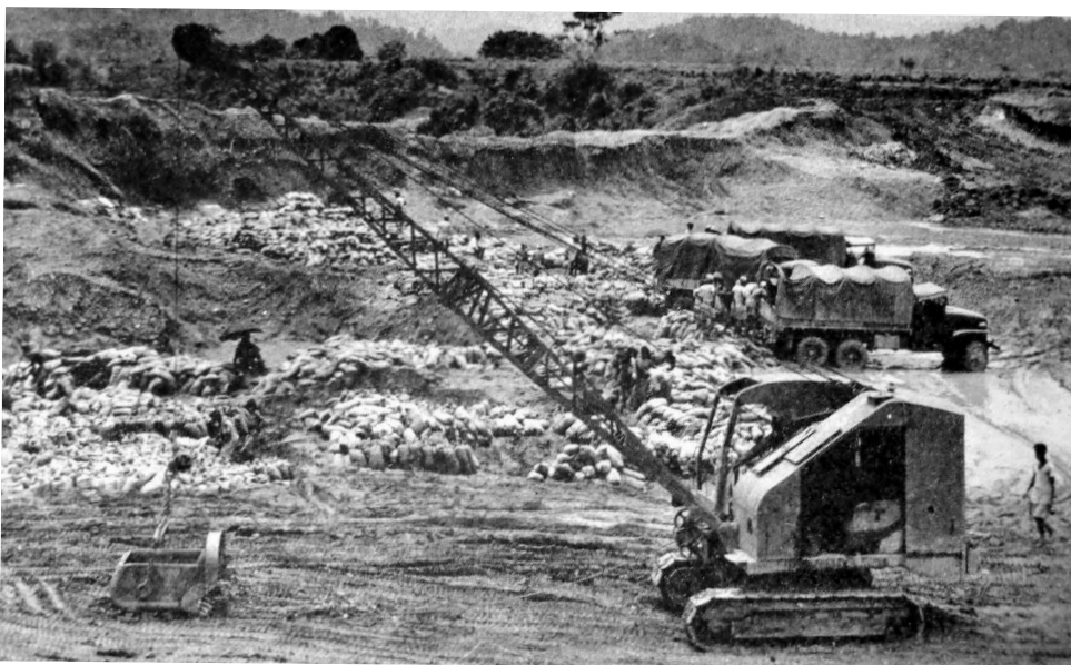
Coolies recruited from tea gardens fill a million sandbags at the Harvey pit for the airport and the Makum Junction Road (1880th Aviation Engineer Battalion).
