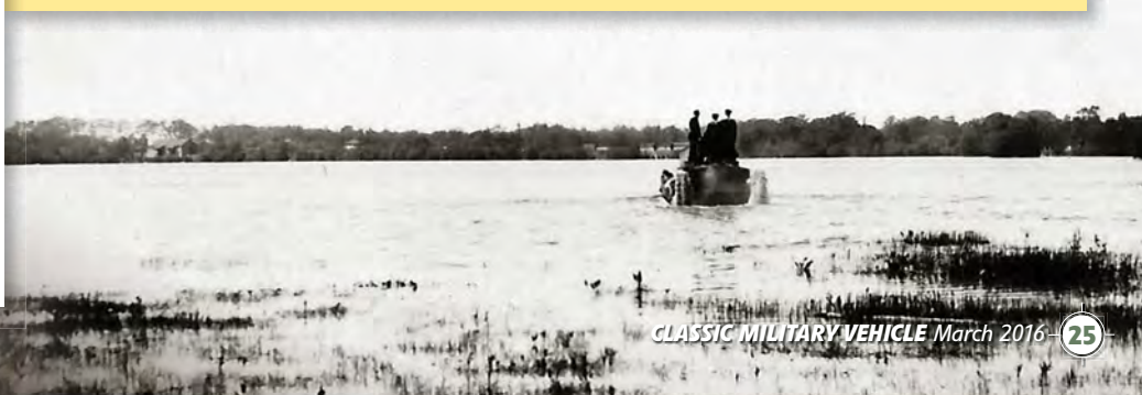
Above: One of the Medium DM tanks undergoing swimming trials. Since they relied on tracks to move them through the water, progress was not very fast. Below: The Light Infantry Tank going for a swim in the Fleet Pond in Hampshire. Obviously the photographer did not want to get his feet wet.
