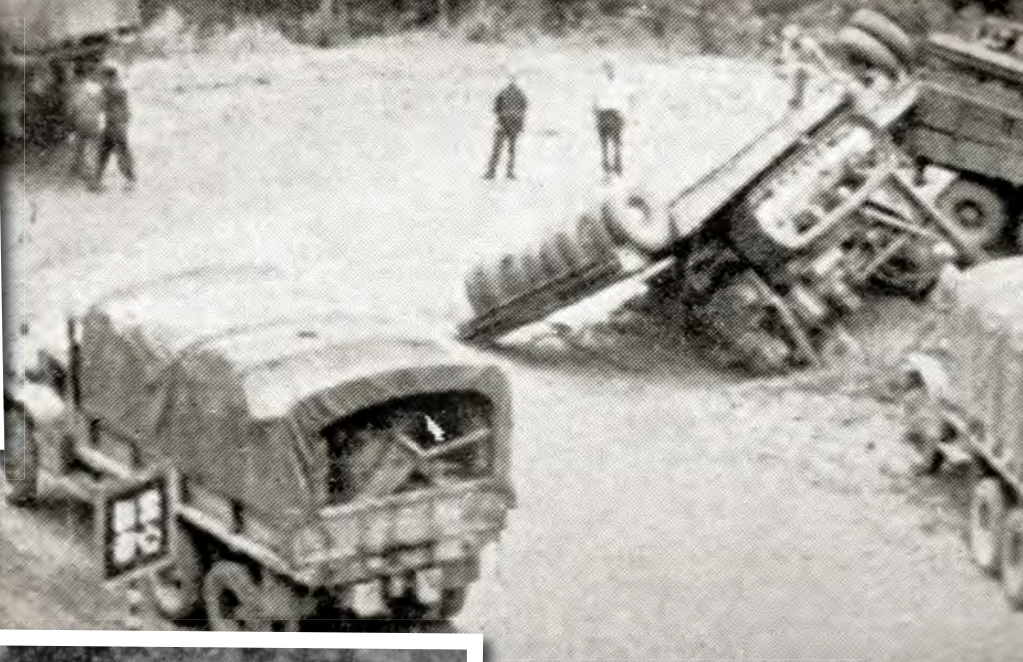
Above, right, below and below right: Example of an accident that occurred sometimes, here near Yang-Pi, China. A Caterpillar D4 has been tipped off on a sharp curve (1880th Aviation Engineer Battalion).
