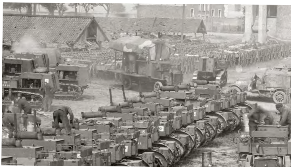
Above: An artillery repair truck FWD is assisting in the servicing of a line of 10-ton Holt artillery tractors. Facing the FWD is a Dodge light repair truck.
