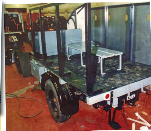
Rear view during the enclosing of the rear compartment with aluminium prior to painting.
