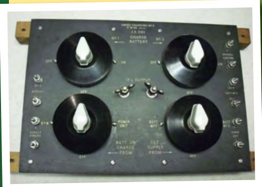
Charging panel enables Jaap to switch between different batteries.
