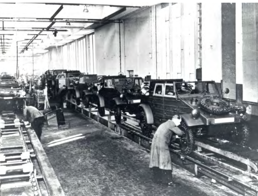
ABOVE: A body drop in the motor-industry tradition mated chassis and coachwork of the Type 82 at Fallersleben. Outside suppliers, including bodies from Ambi-Budd in Berlin, provided much of the initial content
