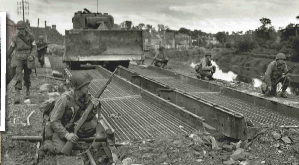
Above: A tankdozer advances across a M2 steel treadway bridge in the Normandy region. Sixteen of the vehicles had been scheduled to land on Omaha beach, but ten were lost before reaching the shore, and one other had to come ashore without the dozer attachment.
