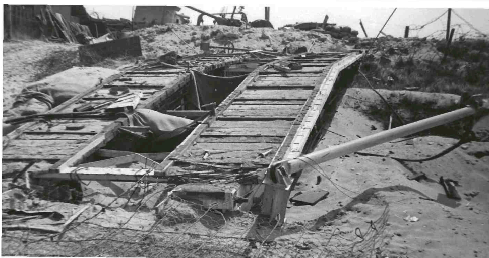
A Small Box Girder Bridge laid across a bomb crater at Lion-sur-Mer. Part of an A frame, lying off to the right shows that this bridge was emplaced by a Mark II, winch equipped AVRE.
