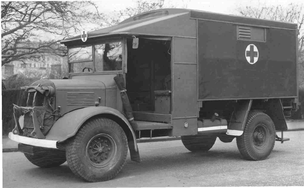
Above: The Austin K2/Y was the largest Allied ambulance of World War II and was used by all of the British services as well as being supplied to the US Army and the Soviet Red Army. More than 13,000 were constructed, with a small number equipped for use as a mobile office or loudspeaker van. (Warehouse Collection) Below: AEC's diesel-engined Model O.853 (and petrol-engined Model 853) Matador was one of the best British trucks of the period. Introduced in 1938, a total of more than 9000 examples had been built by the time production ended in 1945; the majority were equipped as medium artillery tractors. The photograph shows a pair of Matadors, each with a Caterpillar 'dozer load, taking part in the victory parade held in London on 8 June 1946. (Warehouse Collection)
