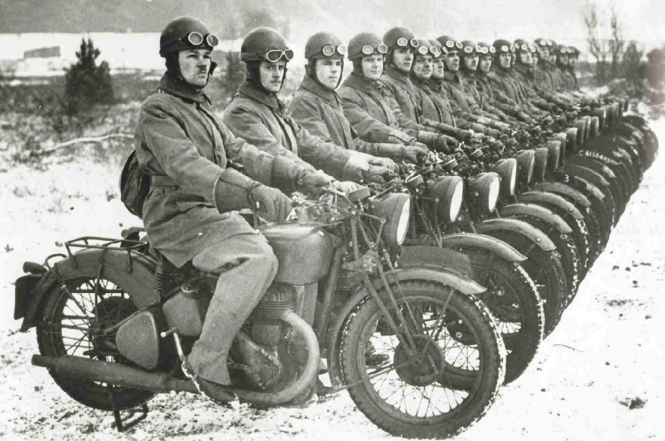
Above: Motorcycles were widely used during World War II for convoy escort work, military police and despatch riders. The photograph shows a line-up of British trainee military policemen, with the rider nearest the camera seated on a 500cc single-cylinder BSA M20. Introduced in 1939, and remaining in production until 1947, some 125,000 examples of the M20 were constructed during the war years. (Warehouse Collection)
