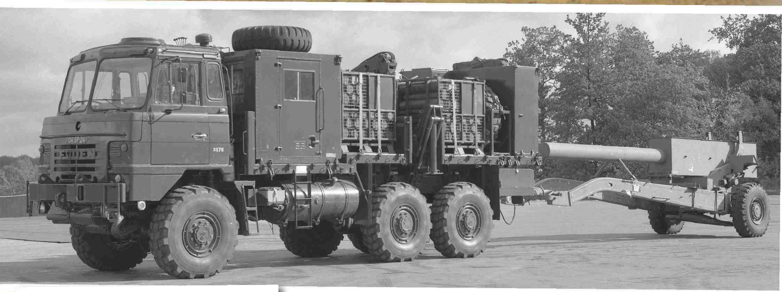
Above: A fully laden prototype FH70 tractor towing a mock-up of the FH70 gun during trials at Chertsey. The mock-up gun appears to use the real trails and wheels of an FH70 and only a simulated gun has been added. (TMB) Left: SP70 was the sister project to FH70. It mounted the same ordnance on a Leopard-based chassis but in a specially built turret. One of its more obvious problems was loading ammunition up to a turret at turret ring height! (TMB)
