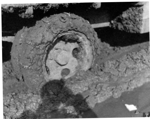
Above left: The performance of road-going tyres was improved by fitting snow chains. A set is seen here, fitted to the outer wheels of a civilian-pattern lorry. They don't seem to have done much good, and may have helped rip up the road surface even more than the tyres themselves would have done.
