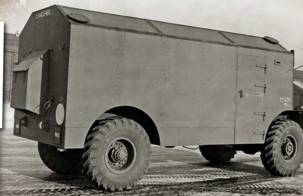
Right: The Armoured Mine Layer variant identified by the fact that someone has helpfully written ML at the front. This type was never developed.
