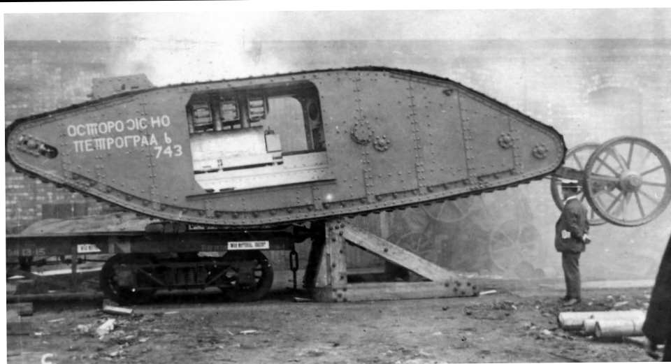
Above: Mark I male tank No. 743 boarding a railway wagon in Foster's yard at Lincoln. It is without its sponsons which haven't arrived yet from Newcastle. 743 was 2nd Lieutenant Bond's tank D18, on the Somme, supporting the 41st Division. Notice the Russian inscription on the front and the clouds of fumes given off by the engine.
