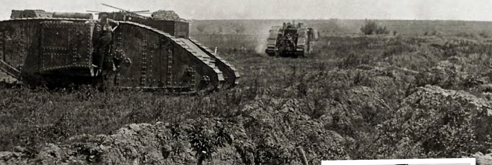
Above: At the battle of Messines in June 1917 Mark Is were reduced to the role of Supply Tanks with their sponsons boxed in and additional stowage trays on top and at the back.
