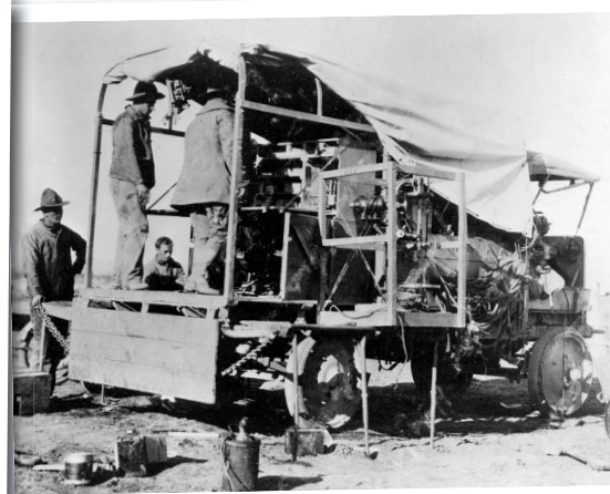
Above: One of the first trucks used by the Aviation Section of the Signal Corps was this four-wheel drive Jeffery workshop truck. The rather primitive open ring gear drive mechanism of the Jeffery suffered very badly in the dusty conditions and many had to be abandoned. Left: Photographed in October 1918 at Beauchamps this Heavy Aviation is towing a stuck British-built Dennis out of a ditch.
