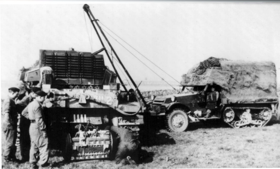
Above: Here you can see the early tubular frame jib from a different angle. This one is in operation in Germany (BAOR). Repairs appear to be the order of the day on this Centurion. Note the extensive camouflage draped over the half-track's superstructure. Below: This photo shows the early tubular steel frame design in operation with its wire supports fixed to brackets welded to the rear of the bonnet sides. This image to my knowledge was taken in Aden and shows the replacing of a Centurion MBT power pack.
