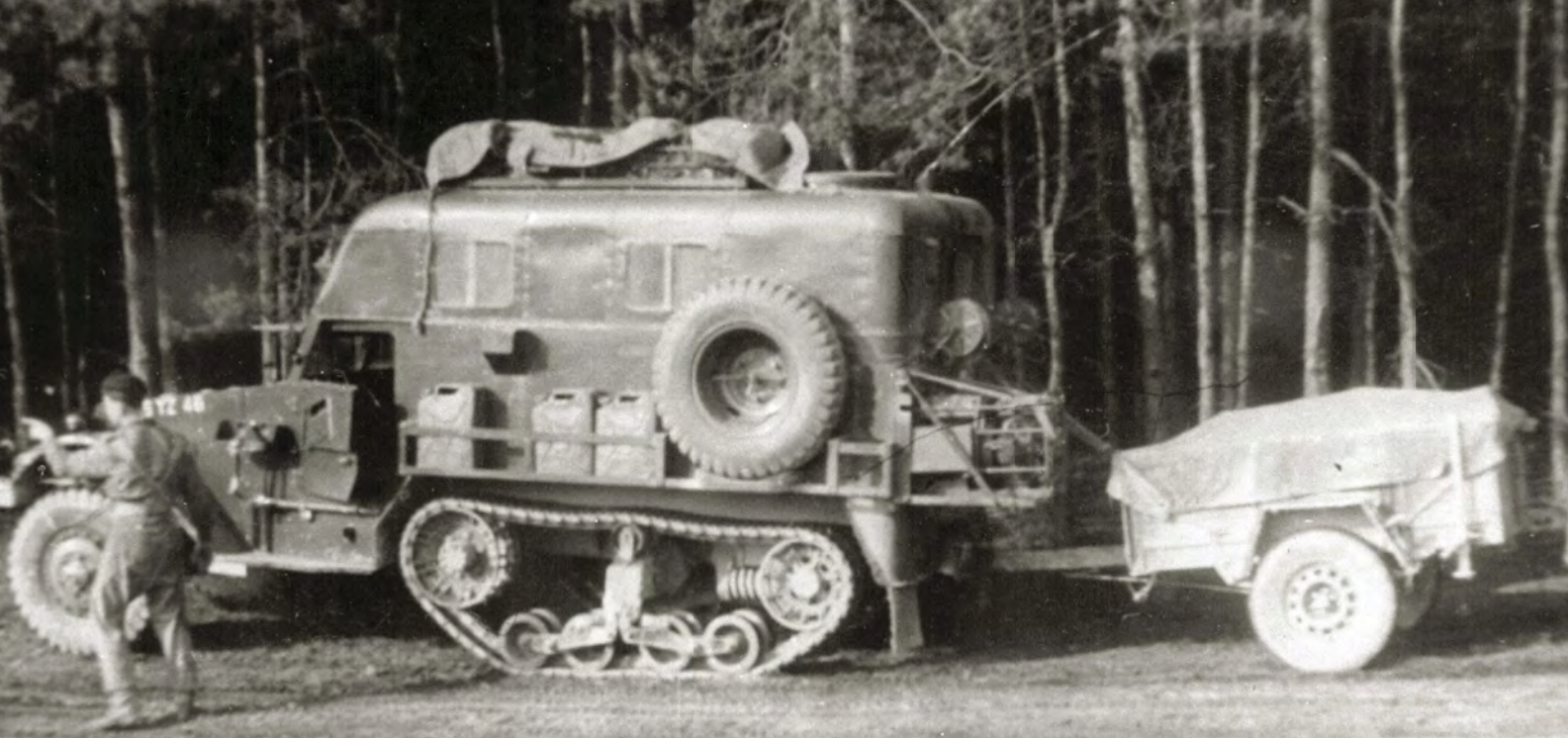
Above: Another image from Germany with a different design superstructure. This one is minus its jib. It is interesting to note the spare wheel has been mounted further back than normal. Fitters vehicles are known to have towed the 1-ton trailer but this one has a WW2 10cwt GS trailer in tow.
