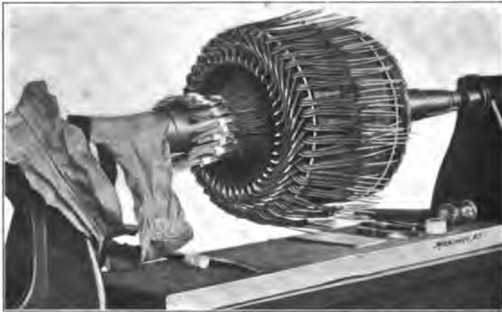
Fig. 66. Truing-up the Winding.
