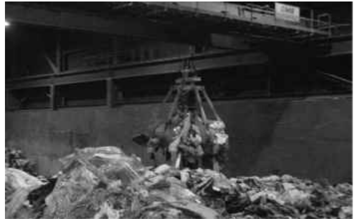
A giant claw moves trash around before it is sent to the boiler. (Pasco County Resource Recovery Facility)
