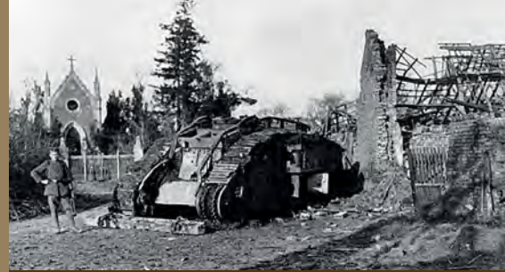
Captured by the Germans is this unidentified MK IV. The wooden un-ditching beam can be seen laying on the ground behind the tank (PHOTO BUNDESARCHIV)
