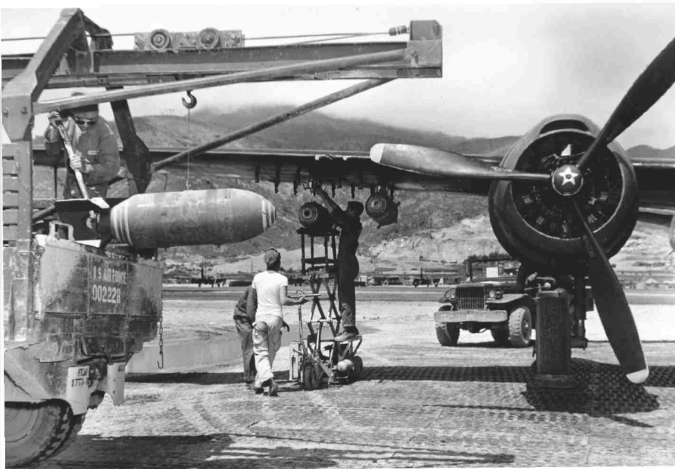
While the bomb trucks were furnished with dollies and tracks, on many occasions it was more efficient to use specialised bomb lifts, as here, to move the ordnance from the truck to under-wing hard points.
