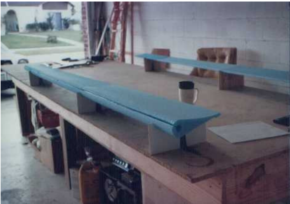
Elevators were jiggled on the flat, level table. Everything needed to be checked carefully for alignment before being glassed.
