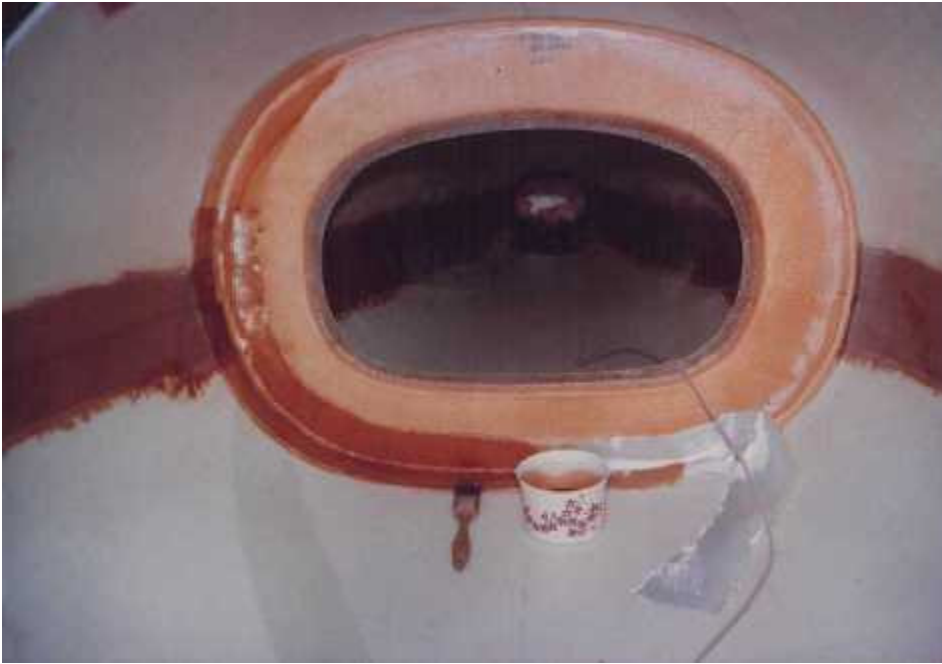
Rear shell bulkhead being glassed in place.
