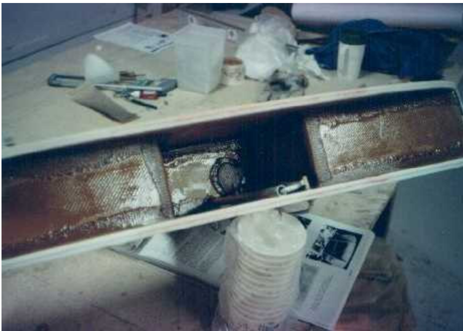
The header tank looking down into the tank.(actually the tank was installed prior to the firewall.)
